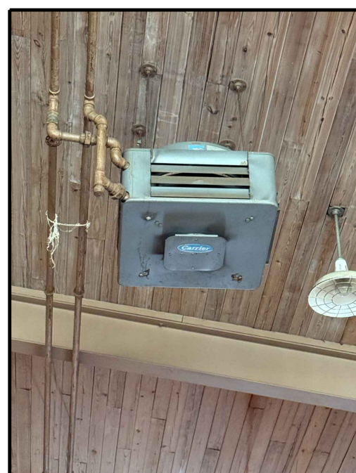
SUSPENDED HEATER UNIT
